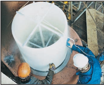
Installation of SXL bearing into housing.
