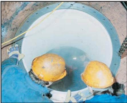
Installation of keeper ring as SXL bearing warms.
